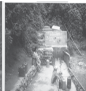
Potable Water Supply
