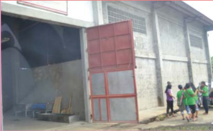
Jagna Common Service Facility for Calamaderas
