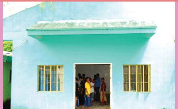
Milaor Common Service Facility
