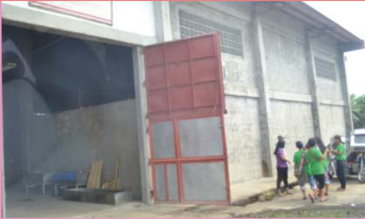
Bula Engineered Bamboo Common Service Facility
